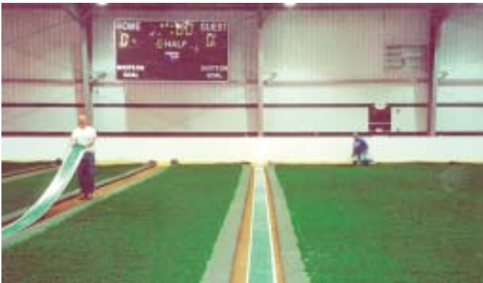
The soccer field under construction.
