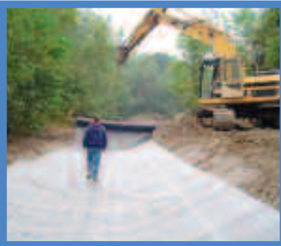
Laying Clay Liner
