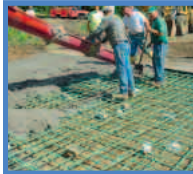
Patching Brass Road
